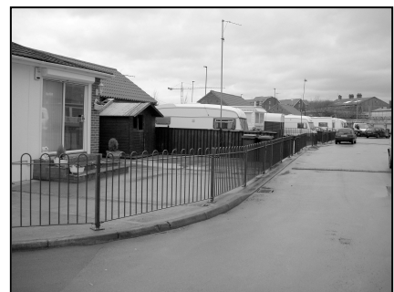
Traveller sites have been refurbished
